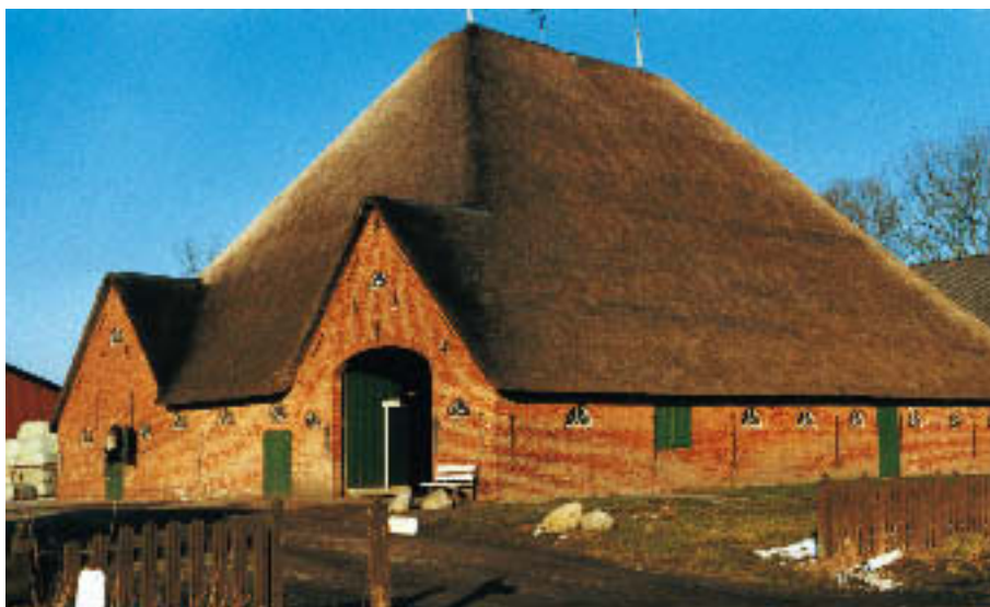
Fig. 4.52: „Haubarg Osterhever“ single „vörhuus“, Barg- construction 4 posts, transformed to a cow-hou- se with financial help for protected monuments
