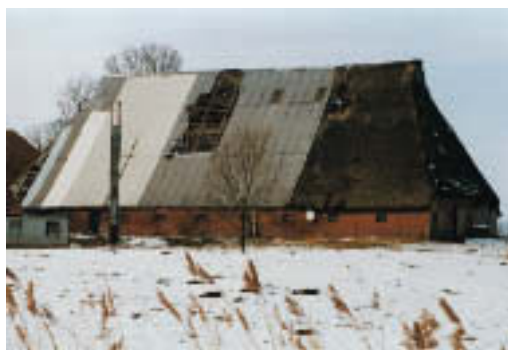
Fig. 4.55: Large „Gulf-barn“ „Siddel- deich“ nearby Hemme, North Dithmarschen No more agriculture, breaking off is possible
